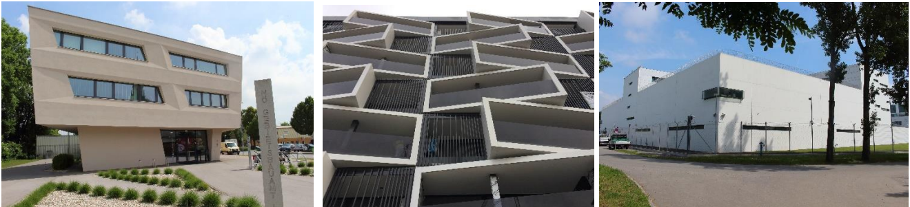
Designs in Passive House construction standard: District building authority (l) and prison (r) in Korneuburg, Austria, © Passivhaus Austria; (m.) residential building in Pamplona, Spain, © G. Velázquez / VARquitectos.
