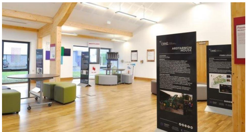
Centre for Renewable Energy and Sustainable Technologies (CREST) in Enniskillen, Northern Ireland: The large areas of glazing at the south of the building assist with solar gain and provide natural light to the exhibition spaces. Information can be found at www.passivhausprojekte.de , ID 5185. © CREST
