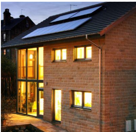
This Passive House in Huddersfield, UK, was the winner of the UK Passivhaus Awards in the category "Retrofit Project". ID 5070 © Morgan O'Driscoll
