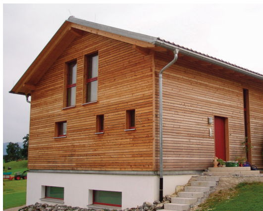
Right: Picture two – Passive House in Steingaden Germany (Herz & Lang project) North-East facades, minimal windows to the North.
